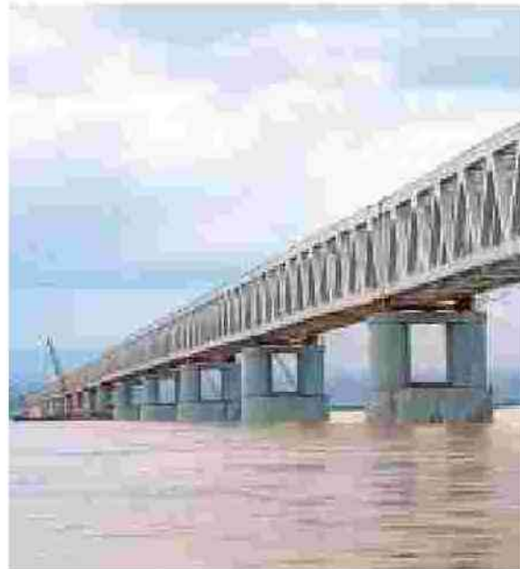
The newly inaugurated Bogibeel Bridge over the Brahmaputra in Assam. ■PTI
