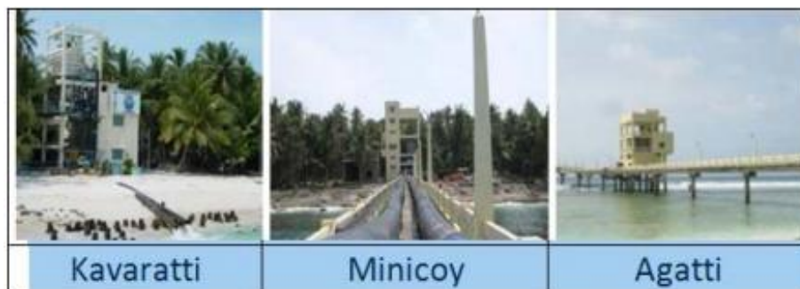
Desalination plant operational in three islands of Lakshadweep
