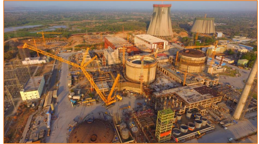
Indigenous Nuclear Power Plant under construction at Kakrapar, Gujarat
